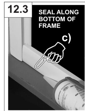
**Do not silicone seal on the inside of unit** (except where shown). Sealing the wallposts & sills to the tray on the inside can result in leakage problems- please note that, in use, water can penetrate into the frame extrusions- *this has no detrimental effect to the product*- however, this water must be allowed to drain out of the extrusions to the inside.
