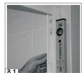
Re-fit clip-in extrusions, which were removed in stage 4. Ensure the leading edge is properly located along full height before pressing the clip-in extrusion into the door frame, it will not locate properly if twisted. *Fig. 9*
