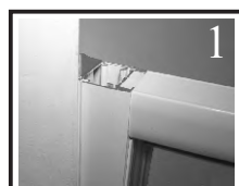
1. Fit connector post cap-push fit.
