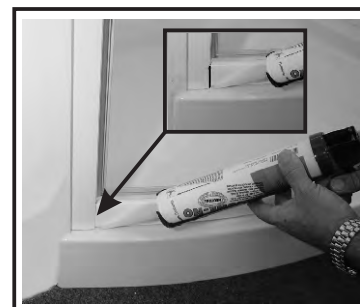
Silicone seal frame to tray and joints as shown on outside only
