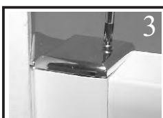
3. Fit top cap screw fix-no.4x10mm csk screws.
