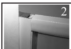
2. Fit channel cap-push fit.
