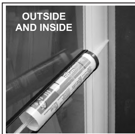
Silicone seal wallposts to wall on inside & outside
